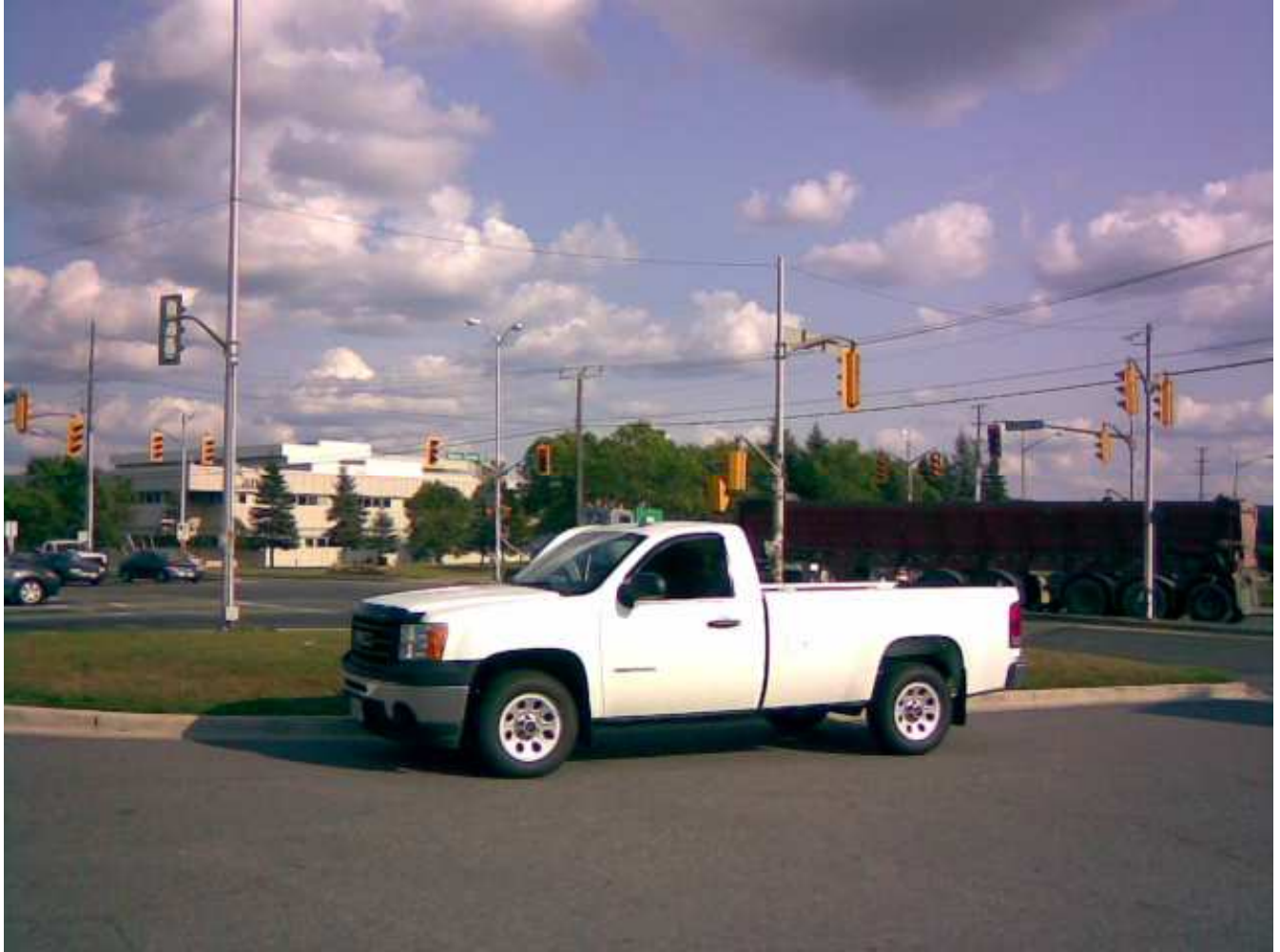
Figure C-1: Lasalle Blvd and Notre Dame Ave – August 4, 2010 (N 46° 31' 20", W 80° 59' 01"). Looking to the southeast
